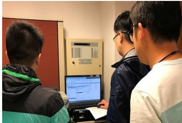
Figure 7 Emergency response mechanism was launched to released weather information during the simulation of communication network failure.
